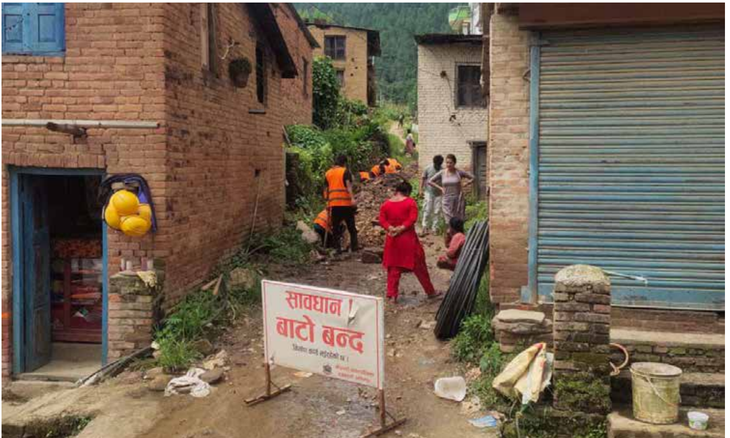
Construction work, Lele
