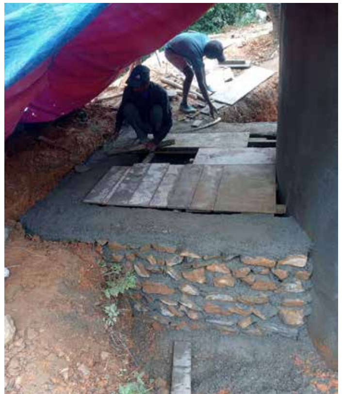
Construction work, Lele
